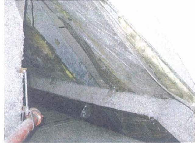
ORD – Chicago Cable Access Level Exterior Wall with Insulation
