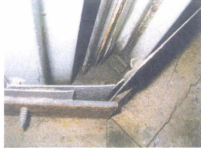
DFW – West Tower Dallas/Fort Worth Cable Access Level Unsealed Walls and Flashing Below Cab Balcony Allows Moisture Into Level.
