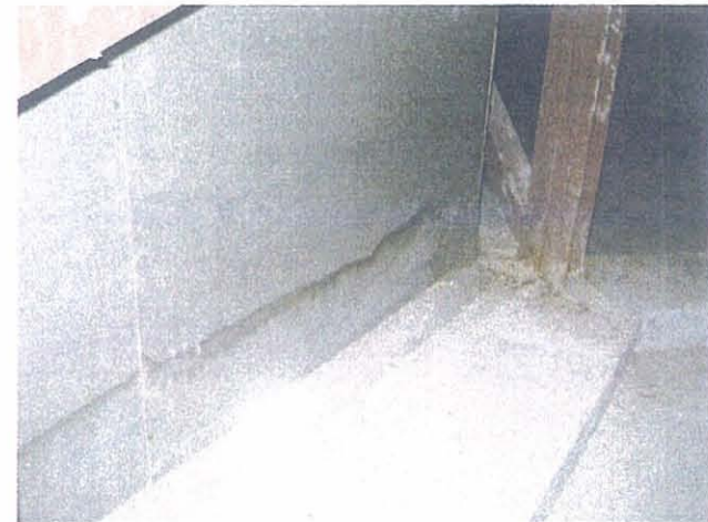
IAH – Houston Cable Access Level Typical Interior Wall
