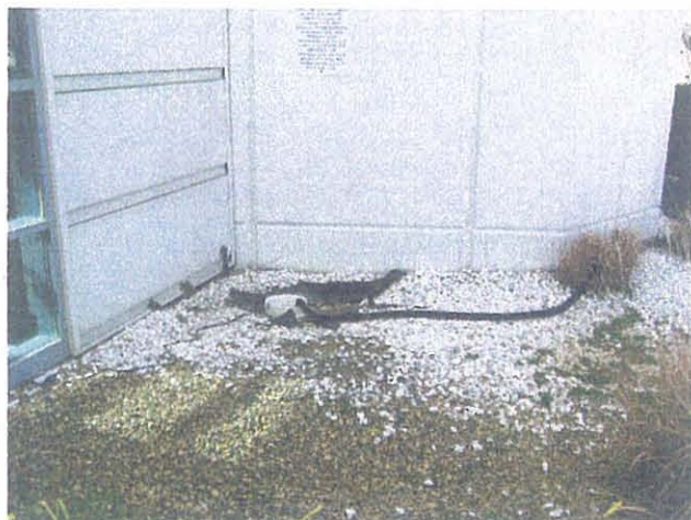
SDF – Louisville NE Base of Tower Makeshift French Drain and Sump Pump
