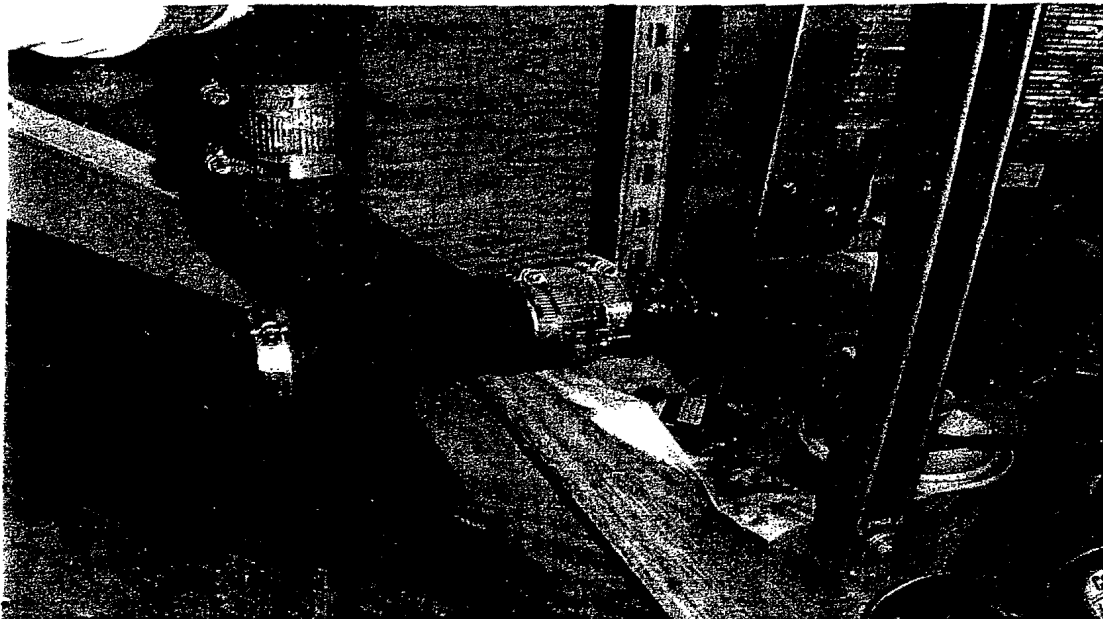
This photo shows the drain line under the Cab sink. The cast iron drain line section shall be removed and cut shorter allowing the cleanout to move to the right creating more space beneath it for a drip pan. The horizontal section of the drain line may also be moved up. A new drain line will be installed from this point to the sink.
