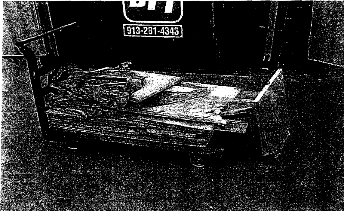
Photo 32: Construction Debris found in 11 th Floor Outer Ring, Back of the West wall of 11TS5.
