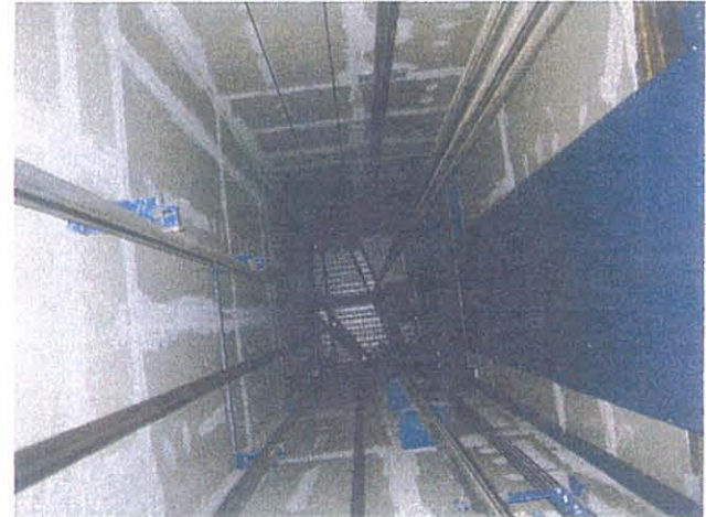
ORD – Denver Elevator Shaft Interior
