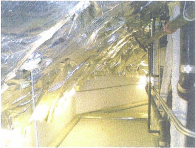
EWR – Newark, New Jersey Junction Level Exterior Wall Insulation
