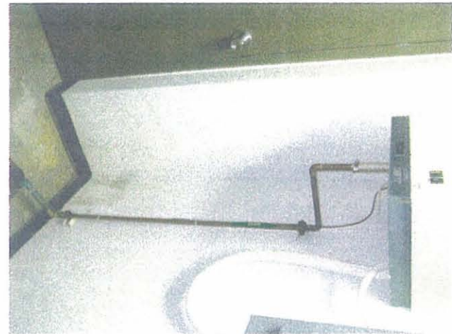
DFW – West Tower Dallas/Fort Worth Cable Access Level Unsealed Walls and Flashing Below Cab Balcony Allows Moisture Into Level.
