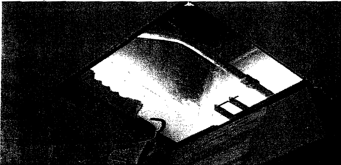
Photo 48: 8TS6 12" by 12" Access Panel Above Ceiling.
