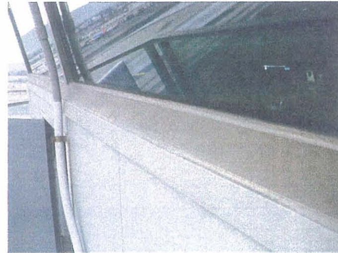
BUR – Bob Hope Burbank Airport Cab Exterior Window Caulk – Good Condition
